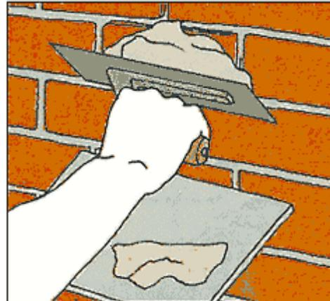
Allow the mortar to slightly harden (2 hours or so) and crisscross score it as shown to a depth of about 3 mm (1/8 inch). Alternatively (if stucco is being applied to a large area) make up a 'rake' by driving a number of nails through a length of 50 x 50 timber at 25mm spacing - make sure that all the nails project the same amount from the timber.
